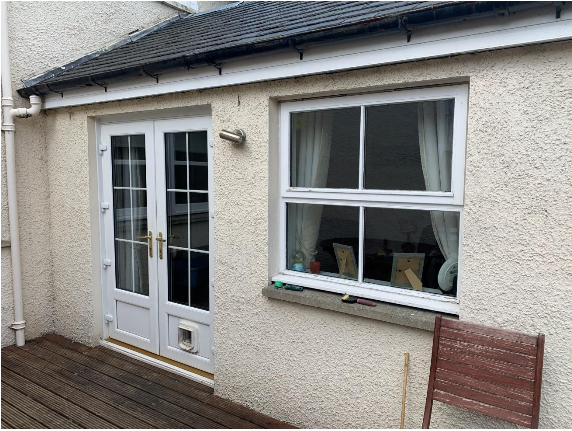
South-West Elevation (Previous extension works)
