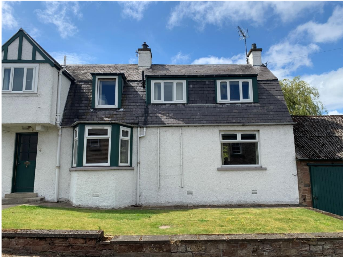
Front Elevation of `Ashlea` (uPVC casement)
