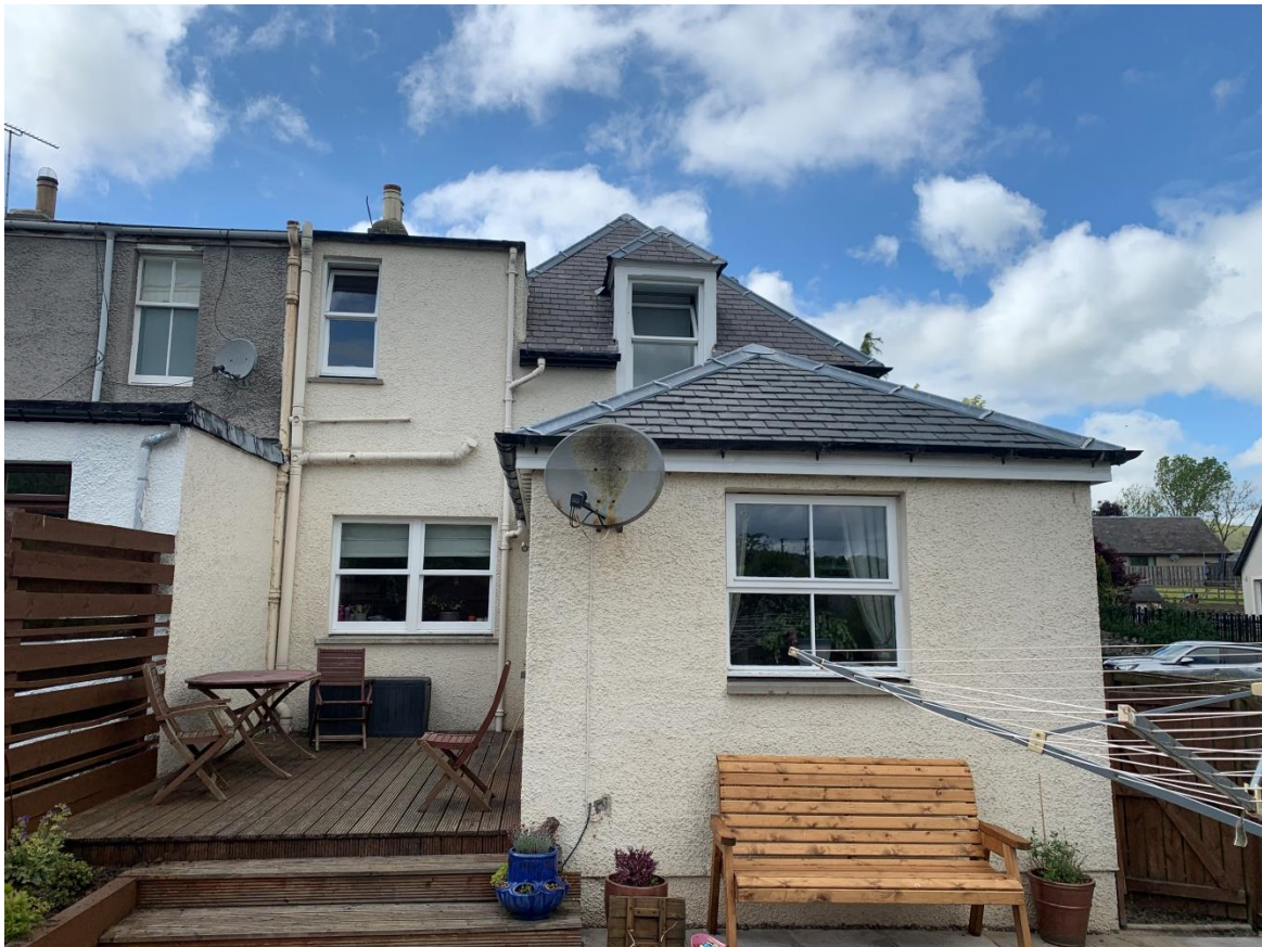
Rear View of House/South-East Elevation
