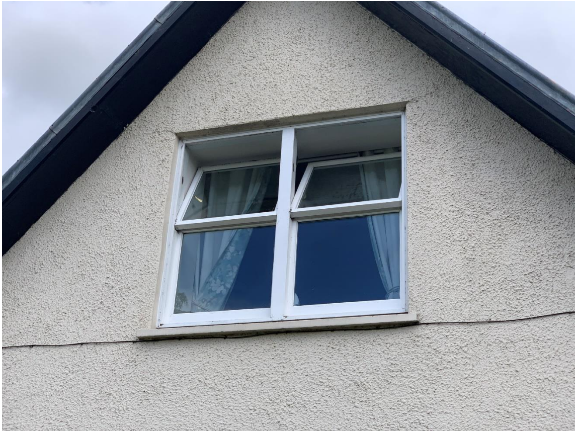
Front Windows (Showing opening style)
